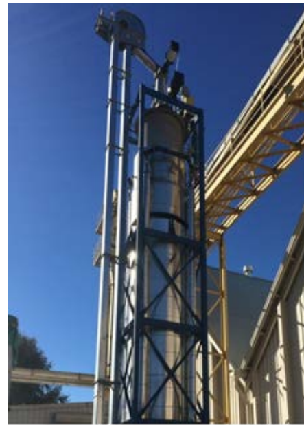
Figure 2: A 2MWth circle-draft biomass gasifier
