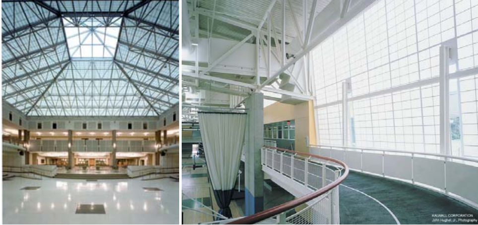
Fig. 5 Two examples of translucent aerogel insulation as a high performance thermal insulation solution for daylighting [35].
