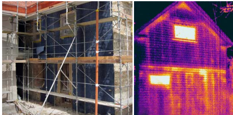
Fig. 6. [left] Aspen aerogel insulation for retrofitting of an old brick dwelling and [right] a thermographic image of a timber wall where the studs of the top floor are insulated with a thin layer of aerogel insulation whereas the ground floor is not [3].
