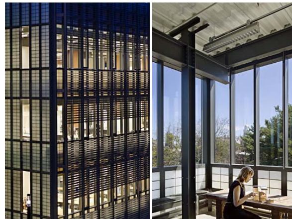
Fig. 2 Translucent aerogel insulation used in a curtain wall at the Sculpture building and gallery of Yale University (New Haven, Connecticut - USA) [77].
