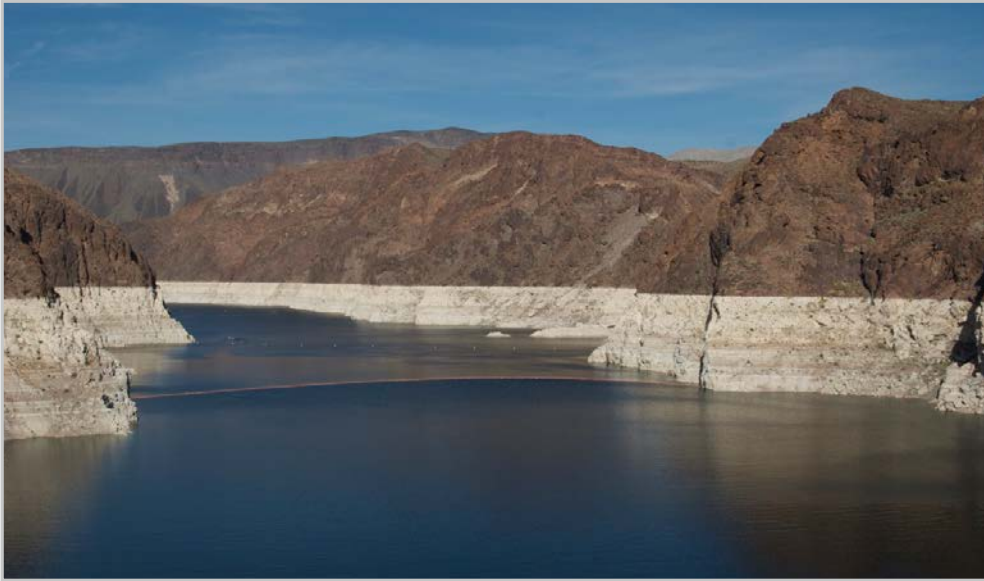
The multipurpose reservoir Lake Mead on Colorado River just upstream of Hoover Dam and Power Plant. The photo is from 2015, close to the end of the 4 years' drought. Photo: Tor Haakon Bakken
