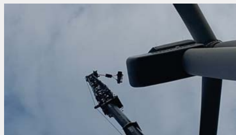
Hoisting the the SpinnerLidar to the Nordex wind turbine at ECN
