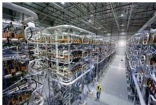
HVDC transmission link between France and Spain: HVDC Plus IGBT converter modules for 1000 MW. www.siemens.com/press .
