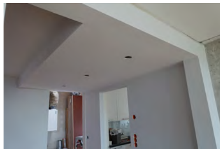
Ferdig himling i gangen
