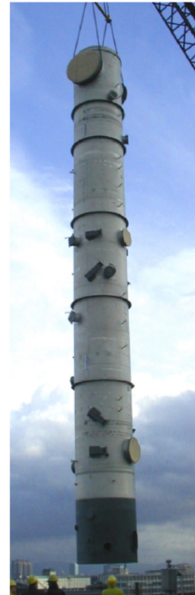
Fig. 3. A photograph of the shell and a drawing illustrating internal configuration of a DWC for separation of a four component feed into pure products.
