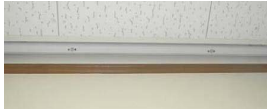
Infrared sensors at each room entrance, which detect in and out of people
