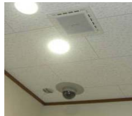
Infrared sensors at each room entrance, which detect in and out of people
