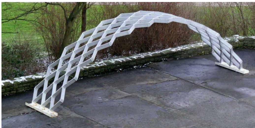
Figure 21: Textile reinforced concrete as a rhomb framework with a span of 10 m. Height and width of each rhomb is 16 cm and 25 mm respectively (Hegger et al 2007)
