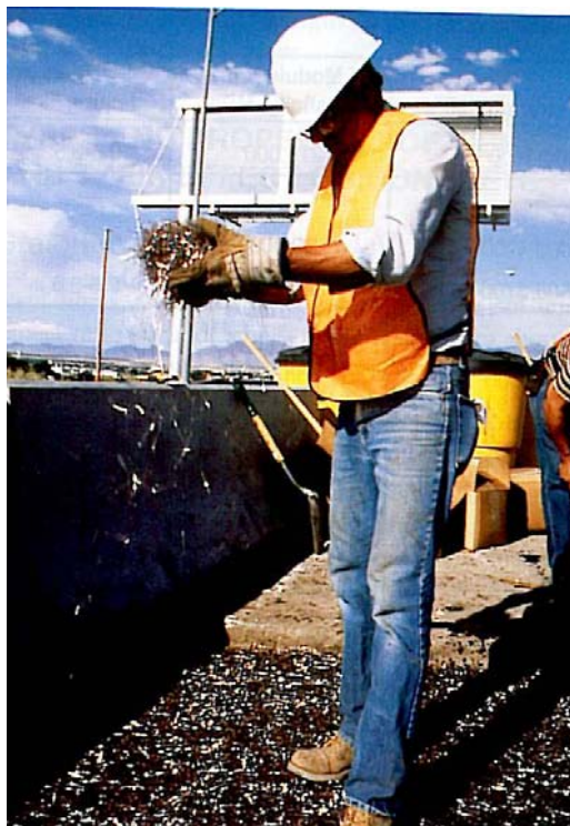
Figure 18: Placing of steel fibres before cement slurry is added in order to produce slurry infiltrated steel fibre concrete (ACI 544.1R-96 1997).
