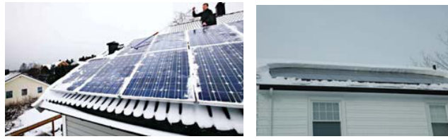
Fig.2. Manual and mechanical methods for removing snow from solar cell roofs (left [15] and right [16]).
