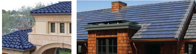
Fig.1. BIPV examples on building roofs (left [9] and right [10]).
