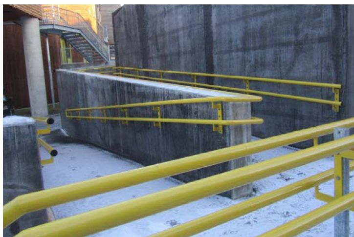
Figure 3: The use of colour on outdoor ramps in Berg student town, Trondheim 2011
