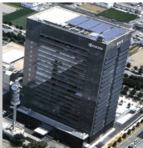
Figur 3.16 Kyocera New Headquarters Building.
