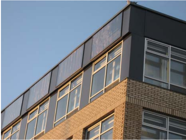
Figure C-9: Solar collectors on the top of the south façade (photo Sintef Byggforsk / Matthias Haase)
