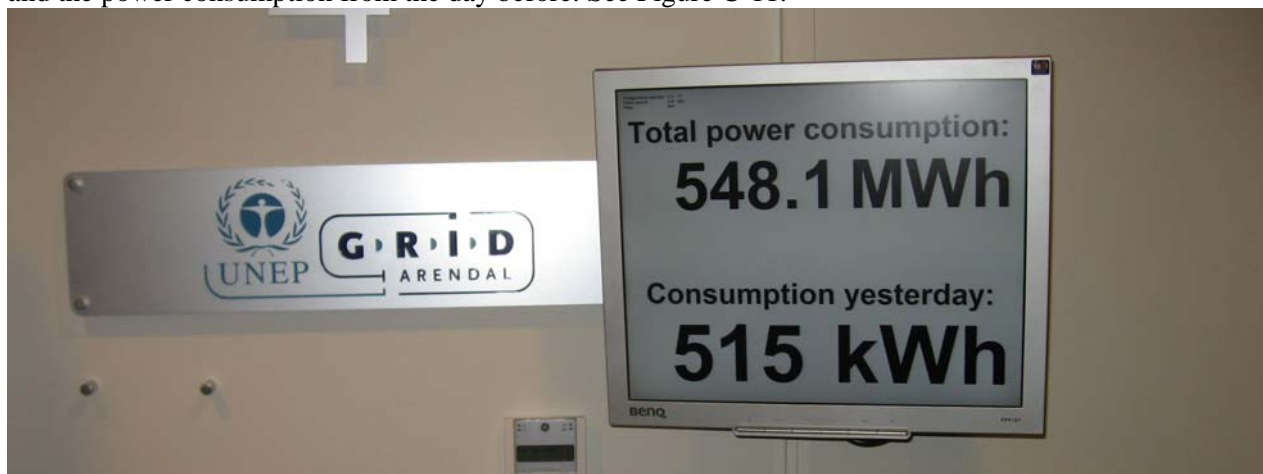
Figure C-11. Display of the power consumption by the entrance of the office area (photo Sintef Byggforsk / Matthias Haase)
