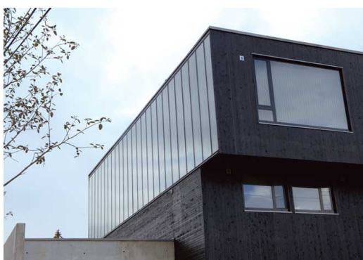
Figur 2.11-2 Plane solfangere integrert i vegg. Foto: Aventa AS
