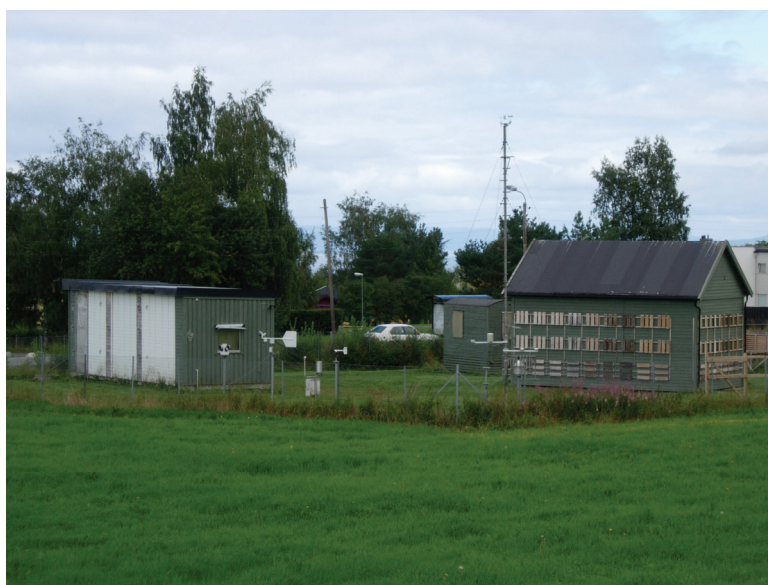
Figure 2.1 An overview of the test station from south-west
