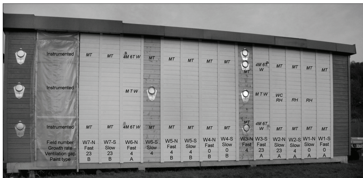
a. West facing wall
