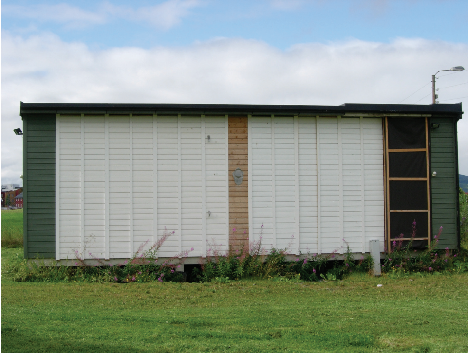
Figure 2.3 The eastern side of the test house.
