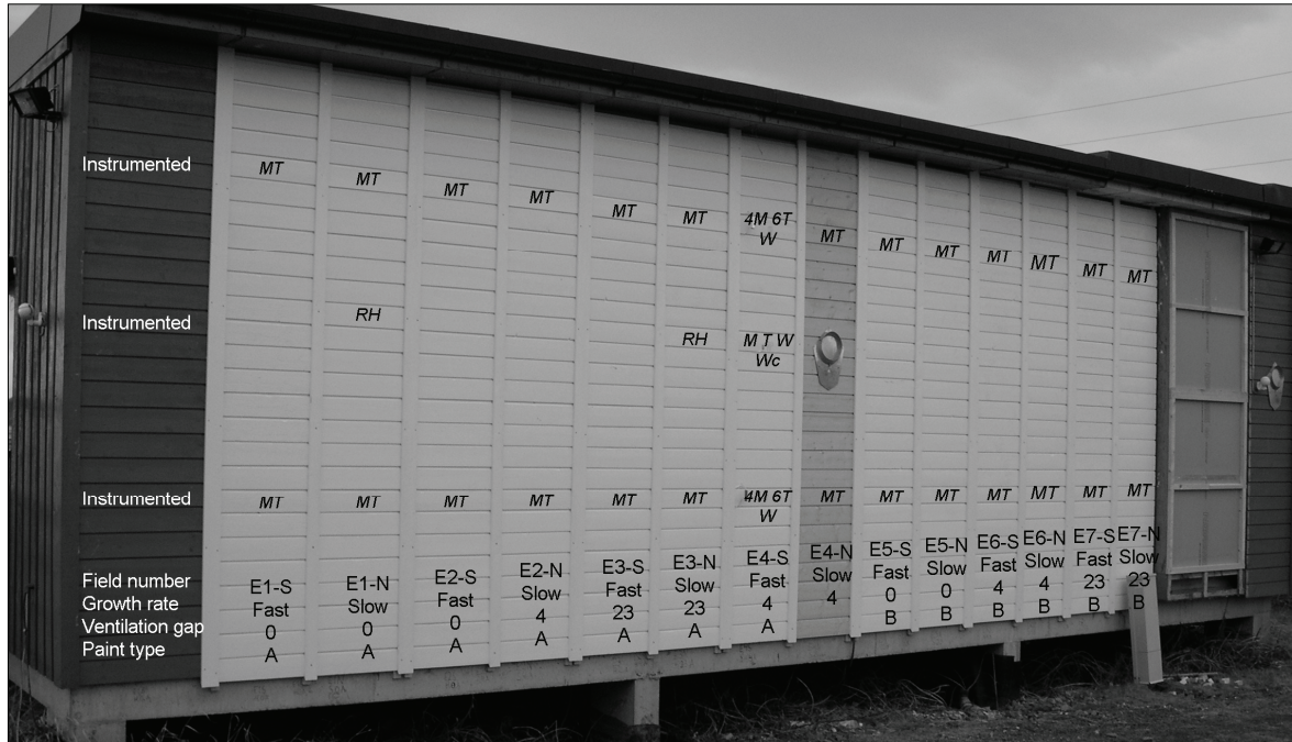
b. East facing wall
