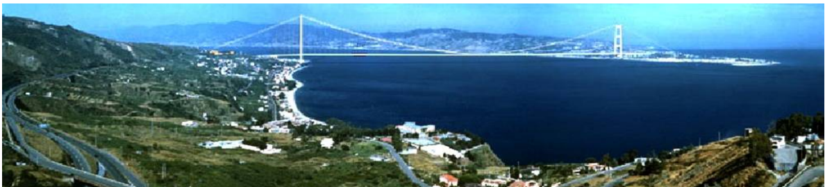
Figure 2-3: Messina Strait Bridge. Design service life is 300 years. Main span in steel is 3000 m. (Model Photo).
