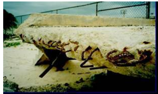
Figure 1-8: Close-up of the land-based remains of the "new" pier as seen on Figure 1-7 /1/
