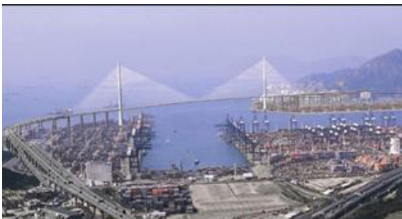
Figure 7-3: Stonecutters Bridge, Hong Kong. Pylons reinforced with SSR (1.4462) in the outer layer of the multi-layer of reinforcement
