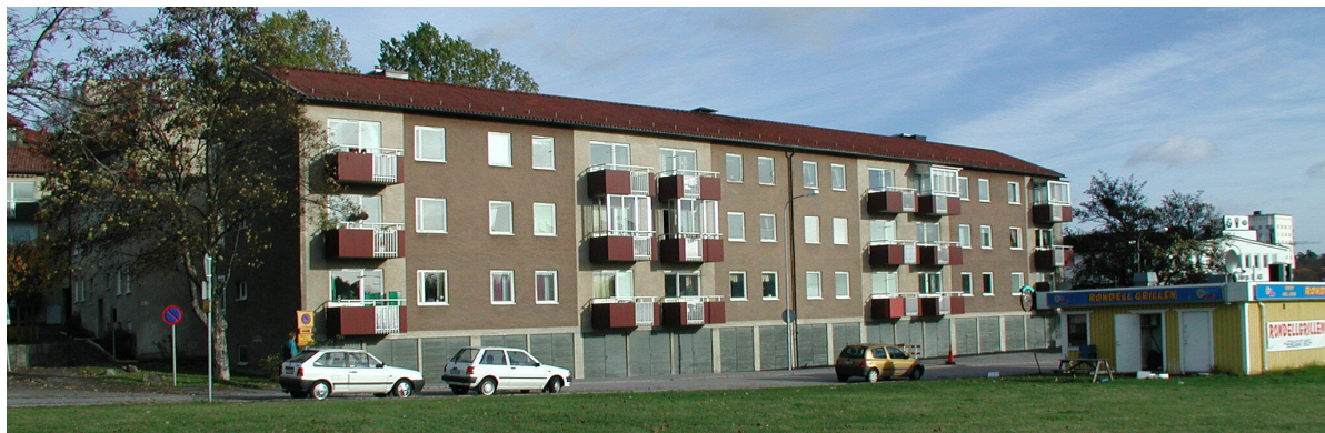
Figure 32: The south facade of the object in Vällingby.
