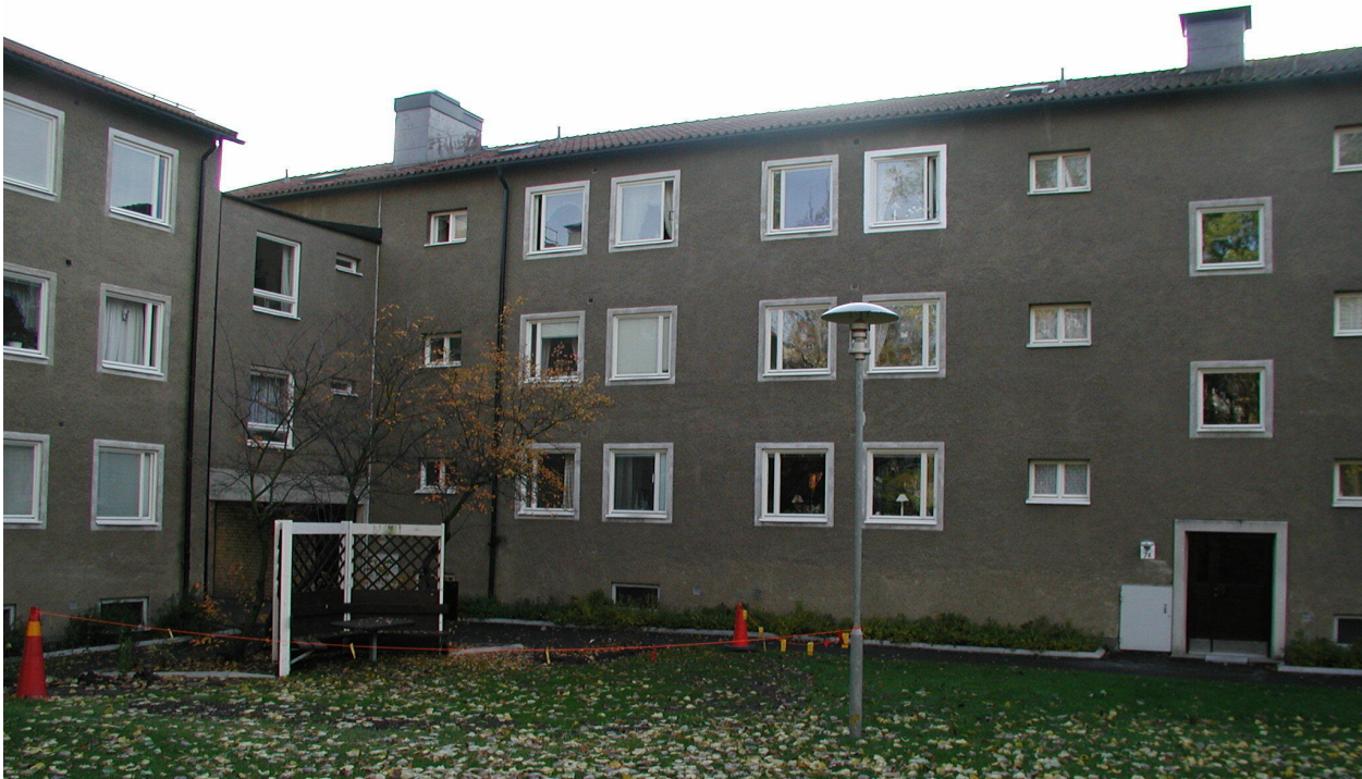
Figure 34: The north facade of the object in Vällingby.
