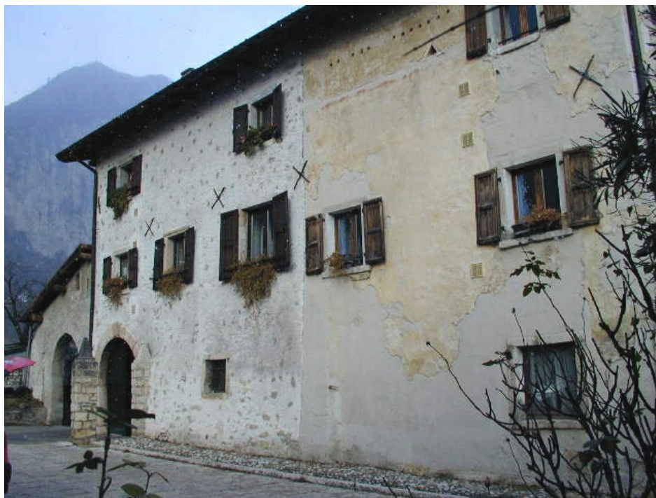
Figure 48: The main facade (south) of Maso S. Cassiano
