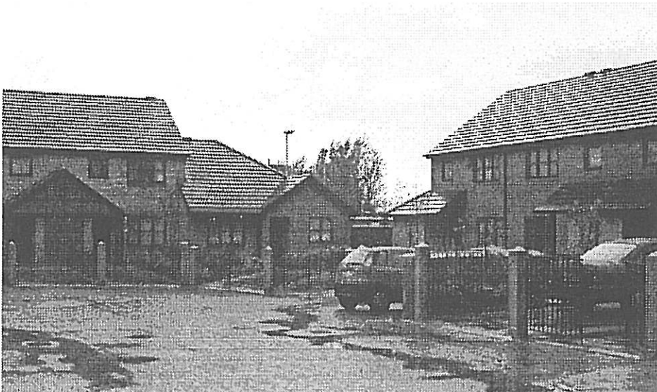
An example of new, two storey lifetime housing that has replaced older tenements on an inner city site in Liverpool.
