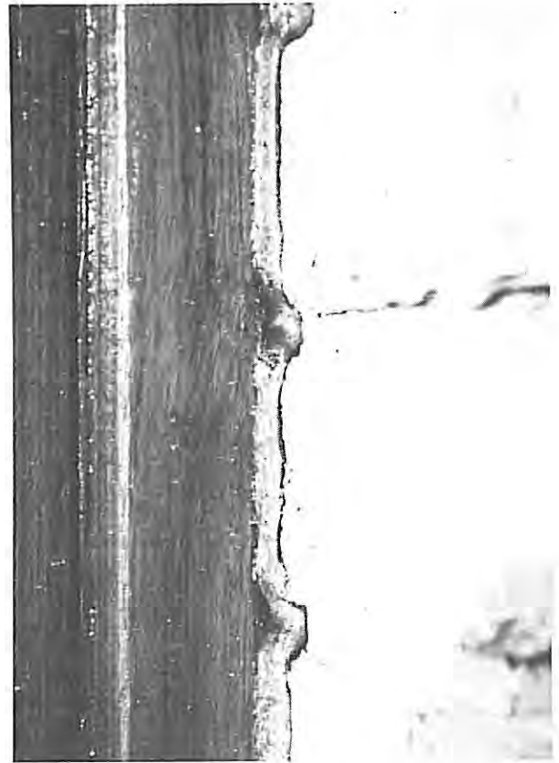
Fig.6. Adhesion loss from a brick wall
