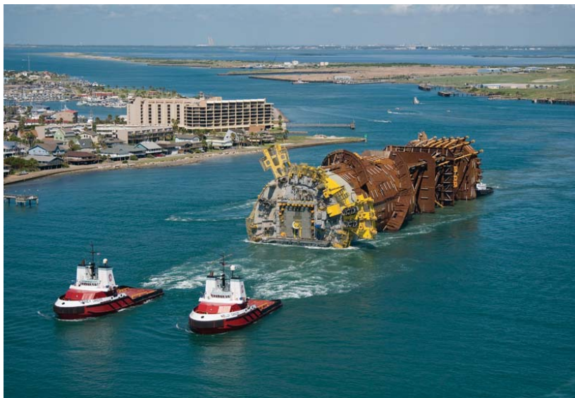
Figure 28: The Perdido Spar during Transport [69]
