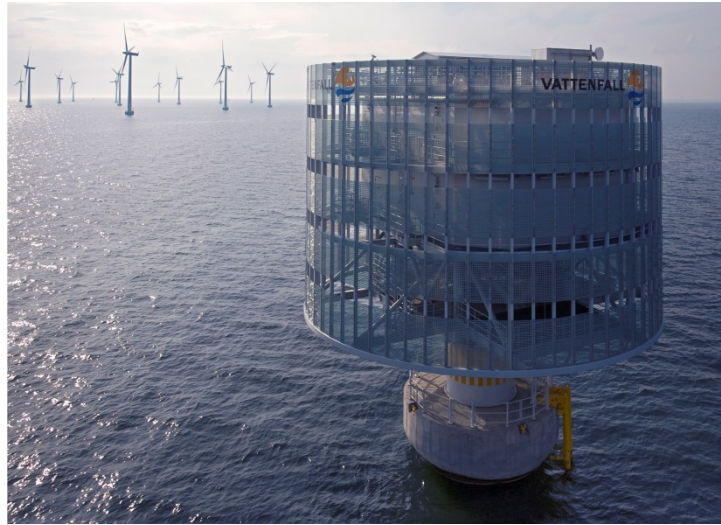
Figure 22: Lillgrund transformer station [62]
