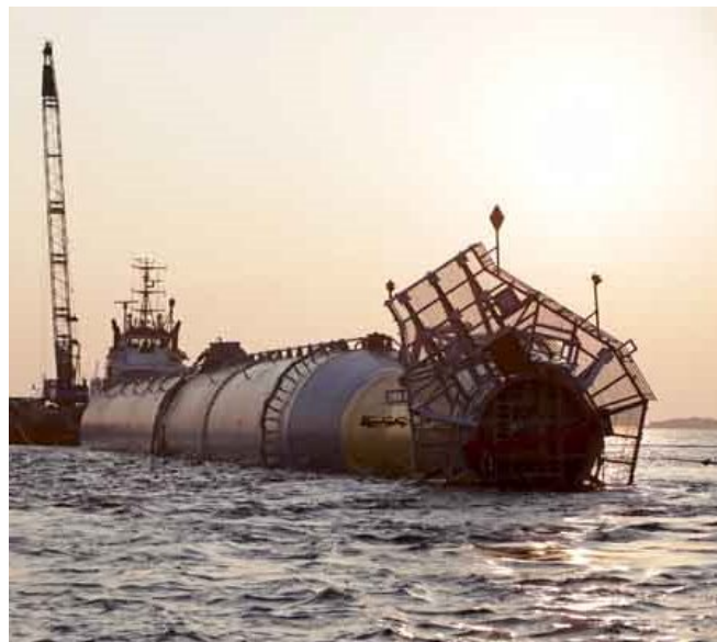
Figure 26: The Hywind wind turbine floating foundation during transport [67]
