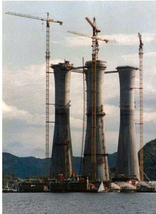
Figure 24: Gravity foundation of Troll A under construction [65]
