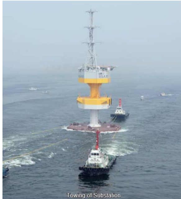
Figure 27: Floating transformer station in Japan [68]
