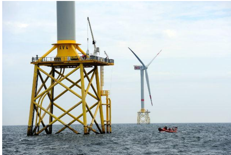
Figure 18: Jacket foundations at Alpha Ventus [58]
