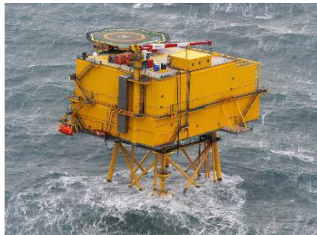
Figure 19: Jacket foundation for BorWin Alpha [59]
