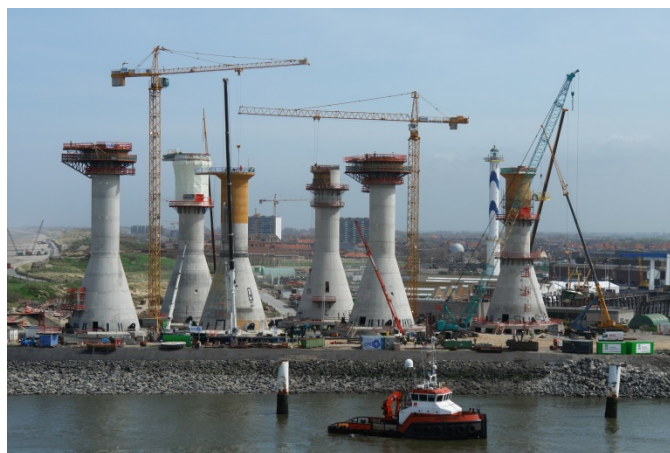
Figure 21: Gravity foundations for wind turbines [61]
