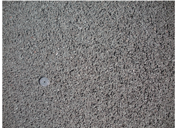
Surface S15: Single layer porous 2/6
