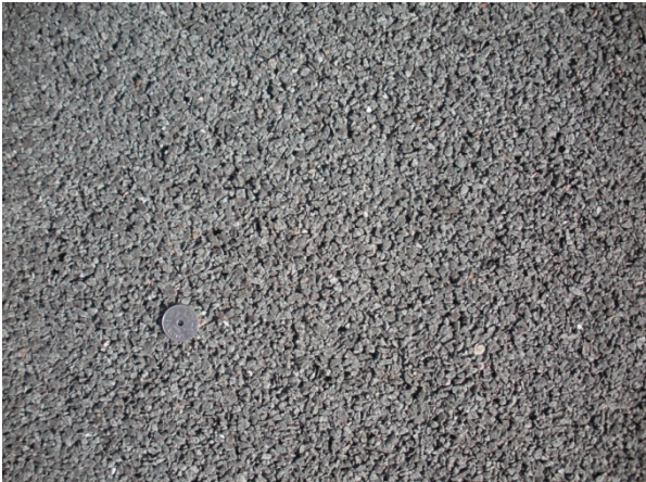
Surface S17: Double layer porous 2/6 + EPAC 0/16
