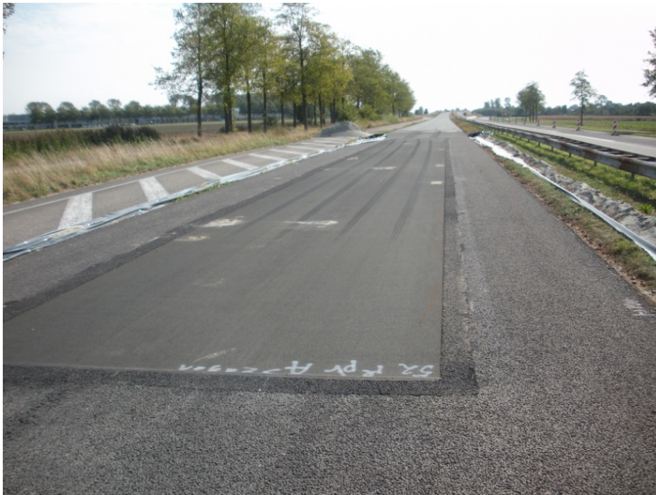
Figure 2 New Rollpave PERS surface at Kloosterzande
