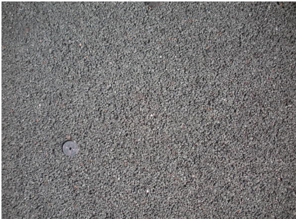
Surface S13: Double layer porous 2/4 + 8/11
