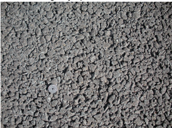
Surface S7: Single layer porous 0/16
