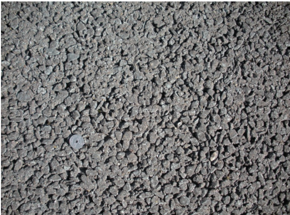
Surface S7: Single layer porous 0/16
