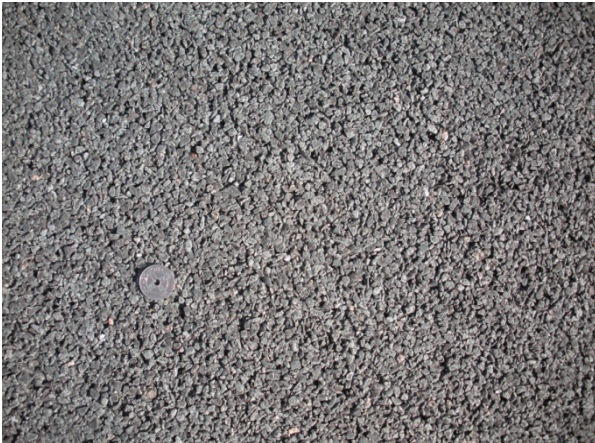
Surface S18: Double layer porous 2/6 + EPAC 0/16
