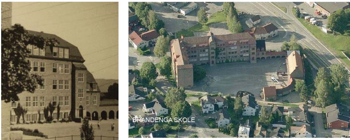
Figure 1 (a): South façade of the main building. Photo from the old days showing the original windows from 1914. Architect Arnstein Arneberg. (b): South façade of the main building showing windows from the 60's and 70's. Note the shading devices. Photo before retrofitting
