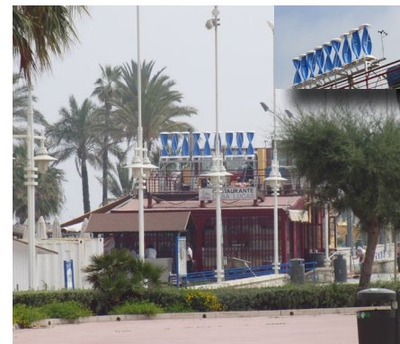
Endesa Install at Casa Lucas: Malaga, Spain June 2012
