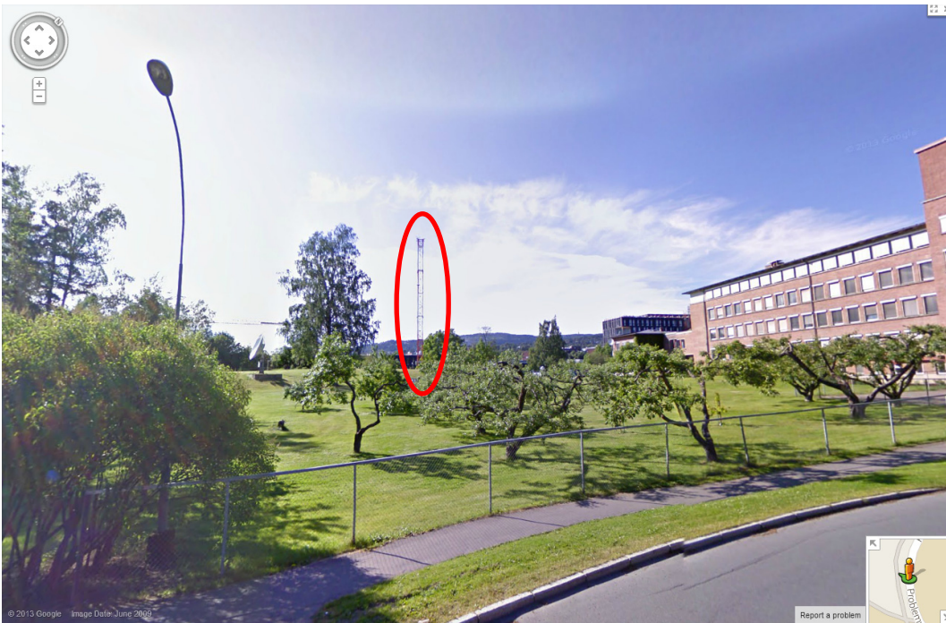
Figure A.6: Weather station Bindern 18700. University buildings and low rise urban environment, looking towards the nearest hill to the north. The wind measurements are taken in 28 m height, due to the proximity of nearby buildings.
